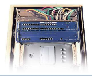
The elmeg ICT series PBX systems can be remotely configured allowing special settings to be undertaken and new firmware loaded directly from your vendor's workshop. This leads to a faster and more flexible service, as well minimising the level of support required. The new PIN concept, which is implemented in several steps, makes it possible to assign individual configuration authorisation sets.
